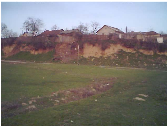
Fig. 14. Erosion at the village border.
