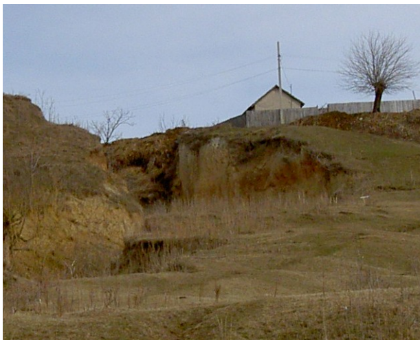
Fig.1 Erosion at the village border in Garla Mare.
